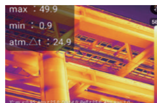
Chemical Operation and Maintenance
